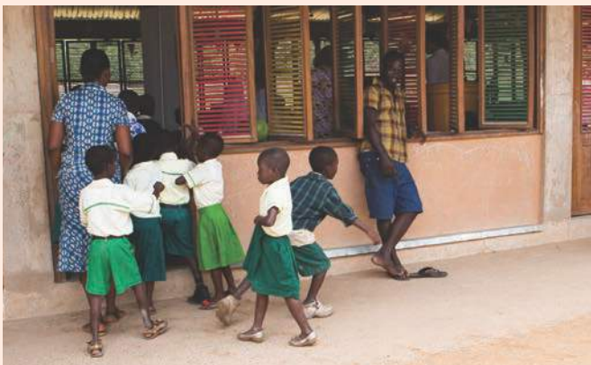
Innovative façade made using pivoting bamboo shutters to allow optimum amount of natural light and ventilation. Photos: Arup & Sabre Trust.
