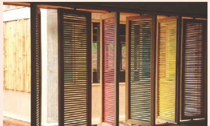
Innovative façade made using pivoting bamboo shutters to allow optimum amount of natural light and ventilation. Photos: Arup & Sabre Trust.
