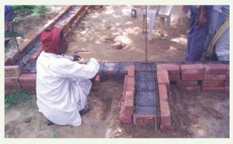
When Uttar Pradesh changed its school design to incorporate seismic-resistant features, the state needed to train masons in the new practices. Five-day trainings that included practice on a mock building taught one or two masons for each new school site how to construct earthquake ring beams in the walls. These trained masons then spread the knowledge to other masons on the construction site. Photo: Sanjaya Bhatia.
