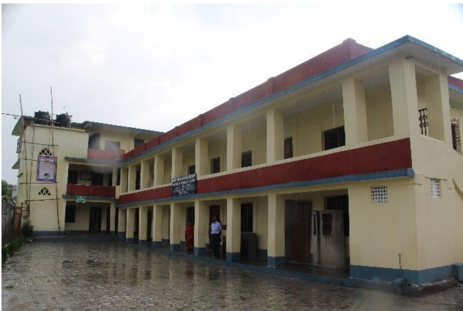
Figure 1. In Nepal, Bal Biskash secondary school (left) was retrofitted through a community-based process. Local masons trained in the earthquake-resistant construction techniques even applied the concepts to local housing repair (right) after the 2015 Gorkha earthquake.
